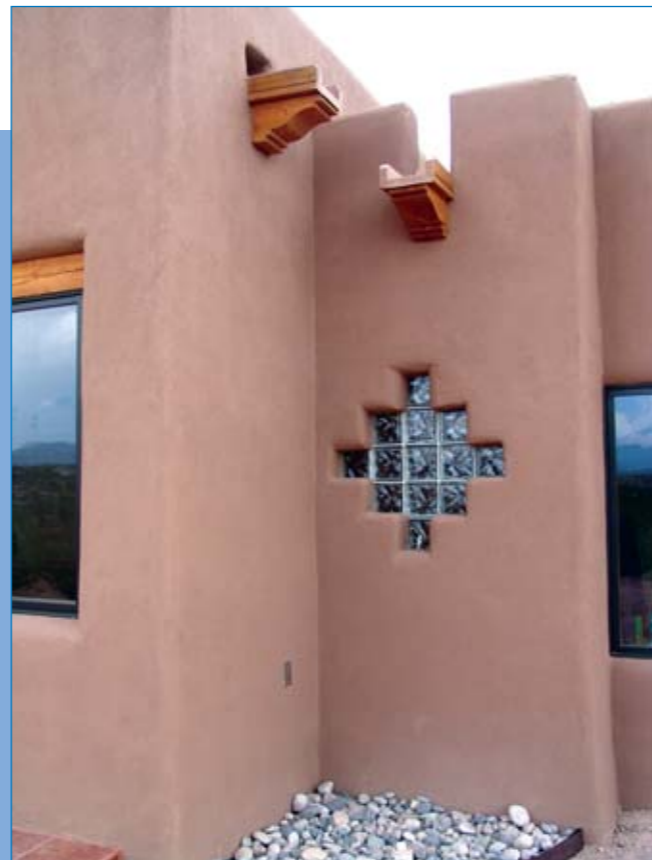
Rain is captured from canals (scuppers) and caught by artificial catchment basin under landscape cobbles. Water is then directed into 4" drainage lines under the surface which transport the water into underground holding tanks, ready for use.
